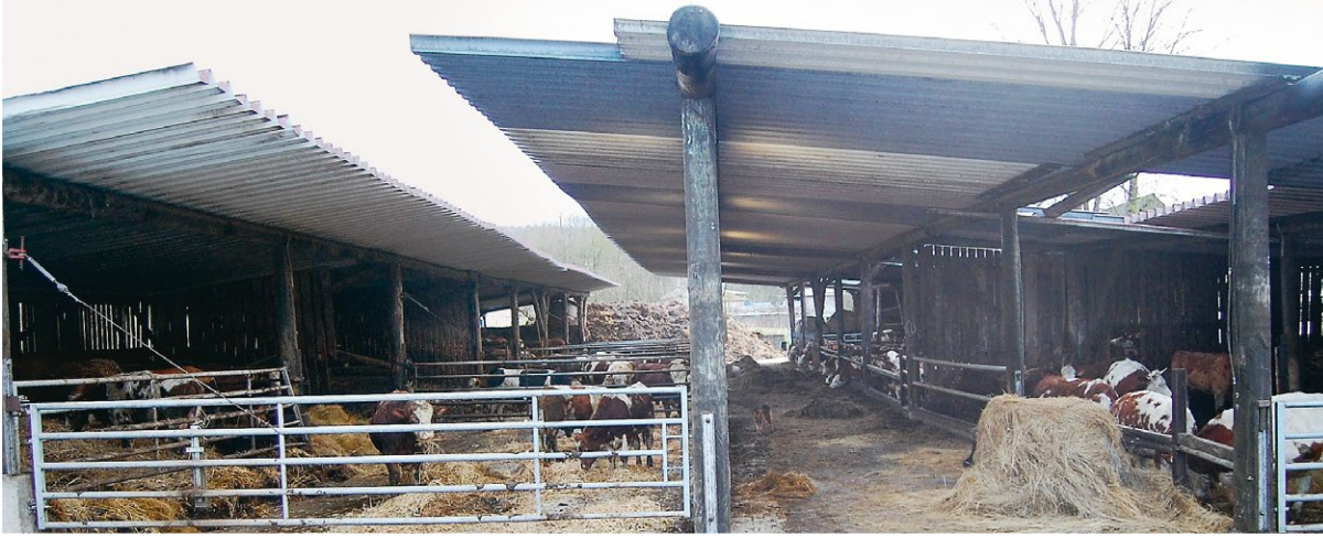
The straw-bedded sloped floor house for the fattening bulls was built in 2006 as a simple round pole construction with monopitch roofs.
