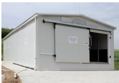
Container dryer with open door
