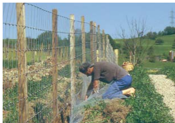
Anti-rodent mesh is being installed along the entire length of the fence. Provisional recommendations for installation:
